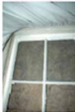
replaced widow frame with modern machined moulding
