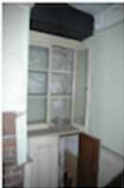
recess cupboards to RIGHT of chimney breast
