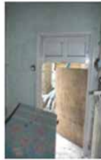
doorway to rear lobby
