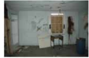
west (window) wall
