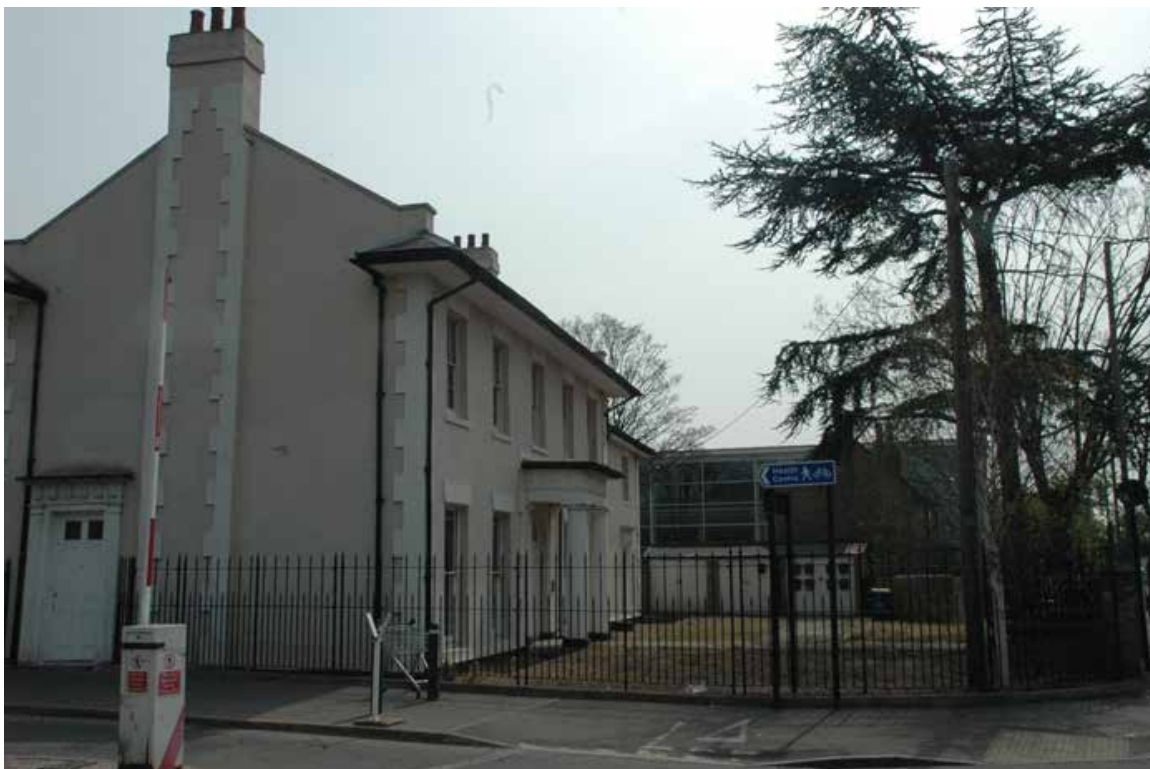
North wall of Thrift Hall looking towards Tesco and Thrift Cottage
