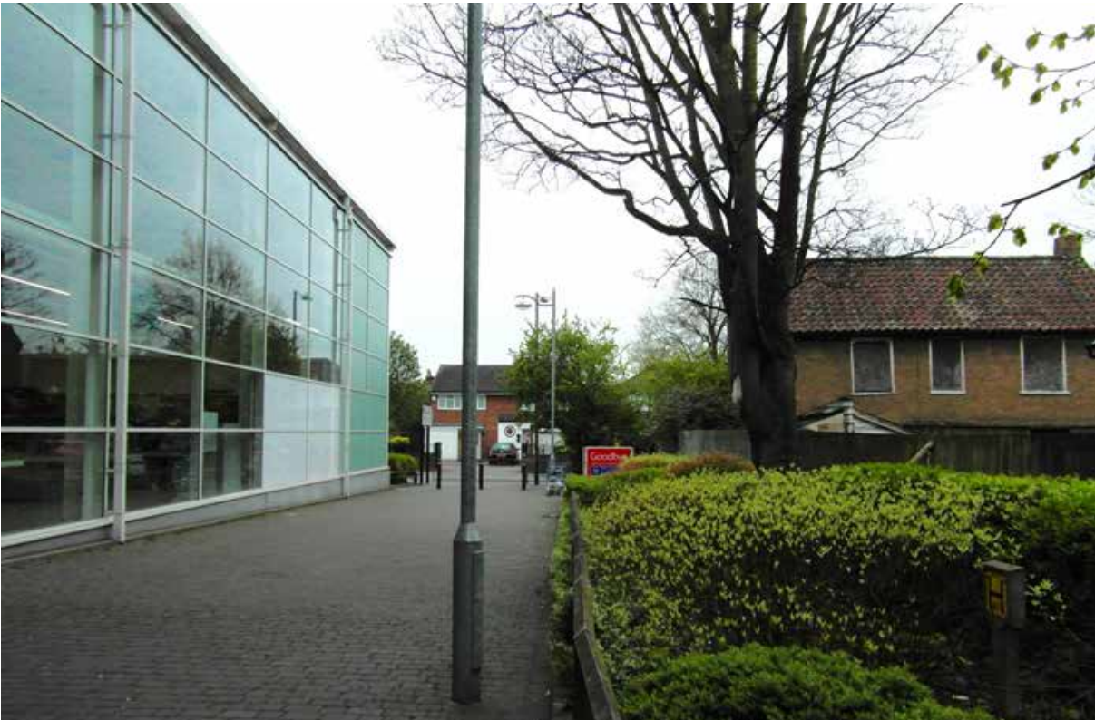
view west along pedestrian paving showing gap between Tesco and Thrift Cottage
