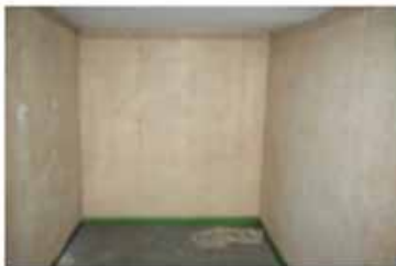
West, north and east walls
