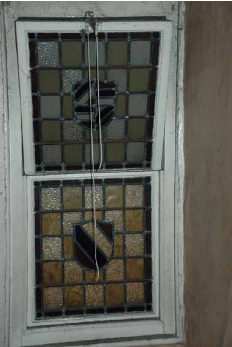
multi-paned staircase window to east wall
