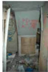
soffit to stairs
