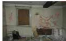
west window wall
