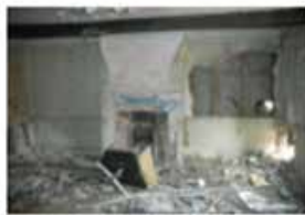
north chimney breast
