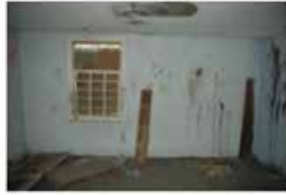
east (window) wall
