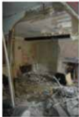
view of n/west corner
