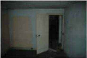
south and west walls
