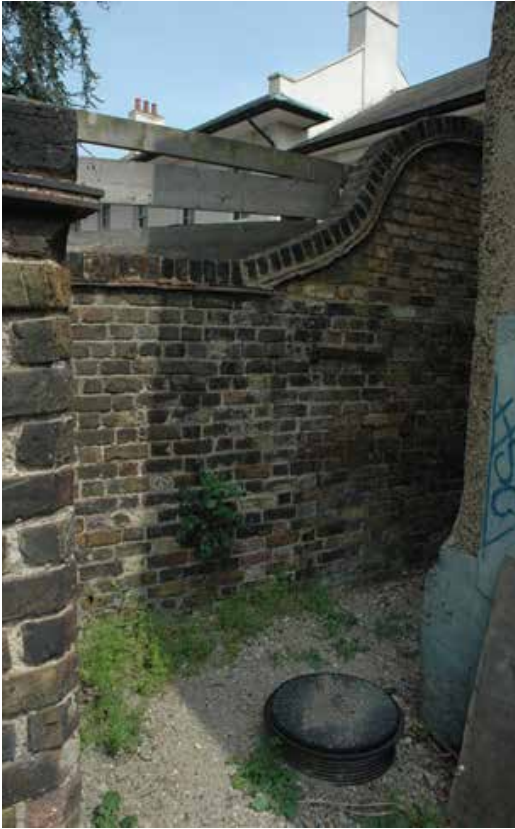
corner of north dividing wall between Thrift Hall and Thrift Cottage
